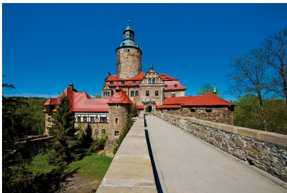
Access path to the entrance
