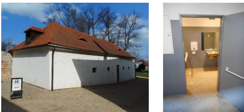
From left: WC building in the castle premises, entrance to the wheelchair WC cabin in the castle premises
